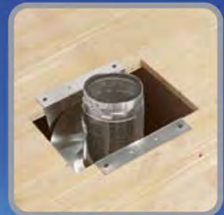
Push pipe through.
