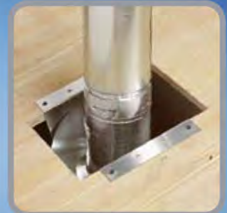
Continue adding pipe sections and termination components. - supports up to 90 lbs.
